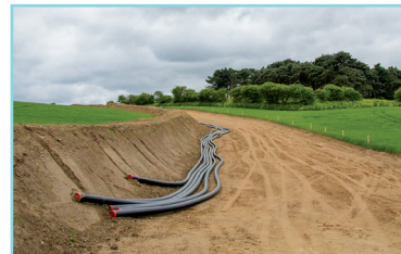
► Cable installation in progress
