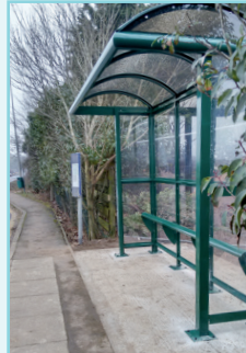
▶ A grant to Necton Parish Council contributed to the erection of two new bus shelters on the A47 highway
