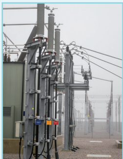
▶ The Necton substation
