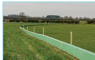
► Fencing to protect Great Crested Newts during construction
